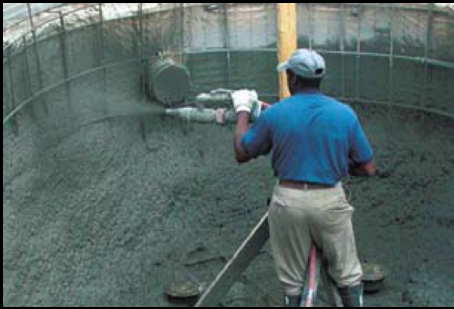
9 mm aggregate shotcrete
