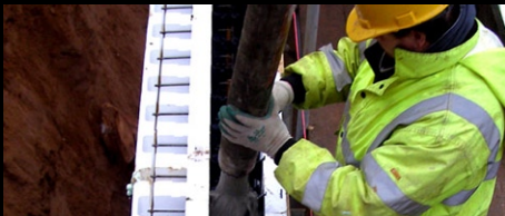
Filling insulated formwork
